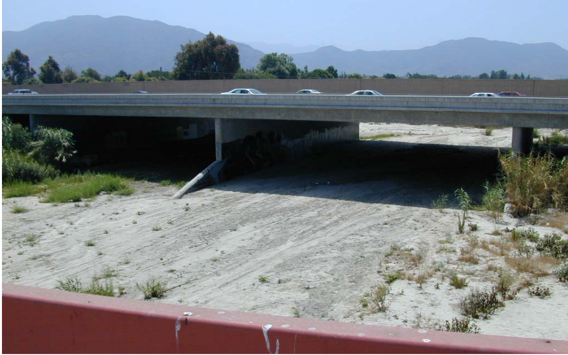
Calleguas Creek at Mission Oaks Blvd., looking downstream at 101 Freeway
