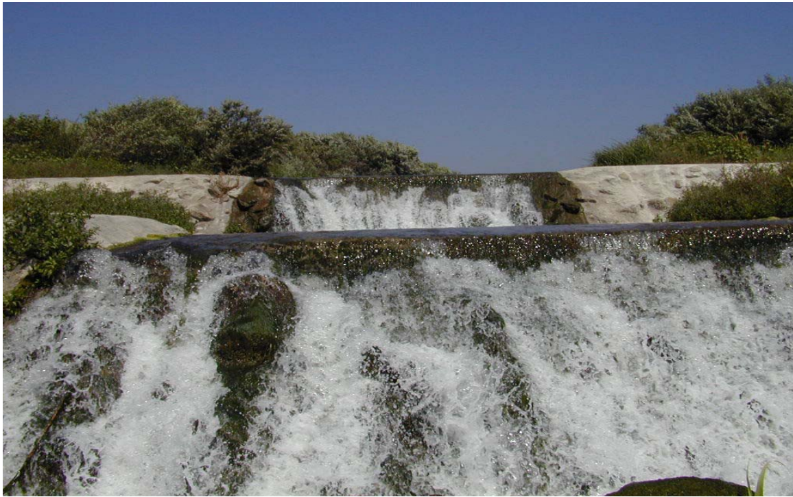
Calleguas Creek at Moorpark WWTP, looking upstream
