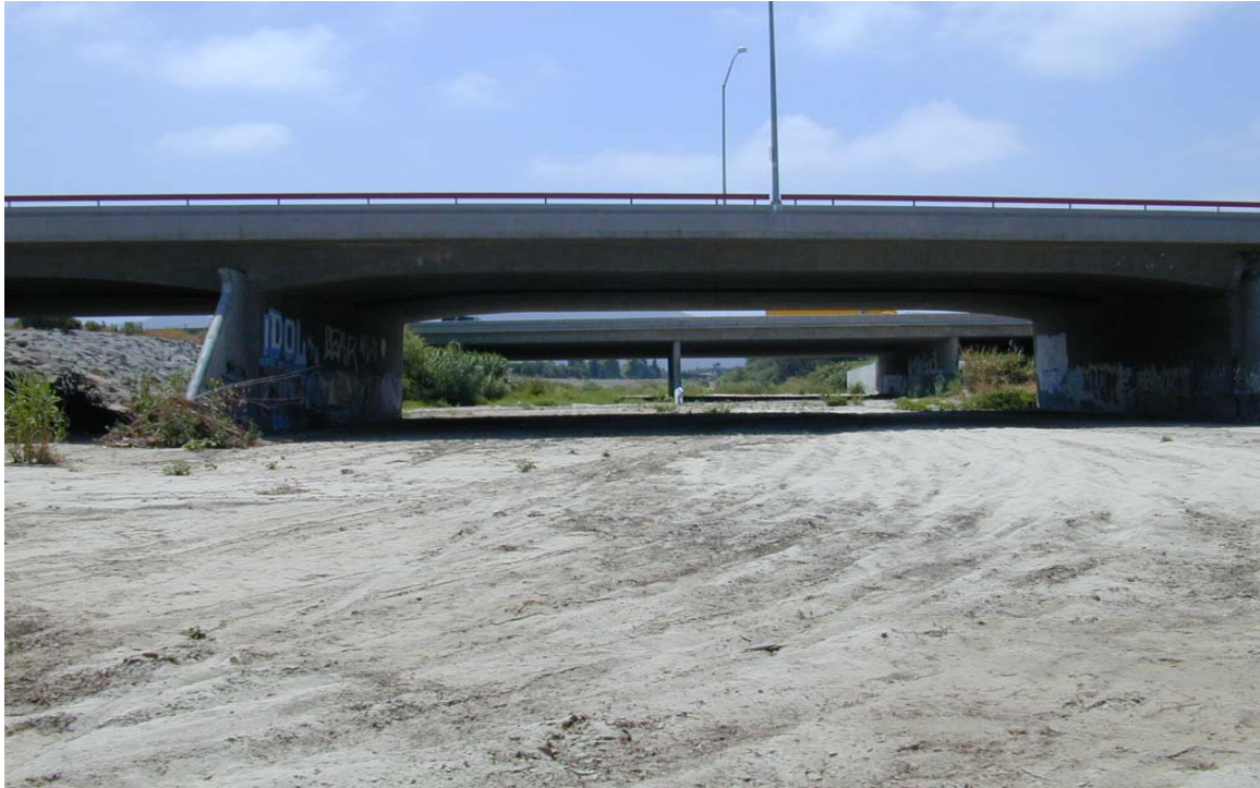
Calleguas Creek at Mission Oaks Blvd. and 101 Freeway, looking downstream
