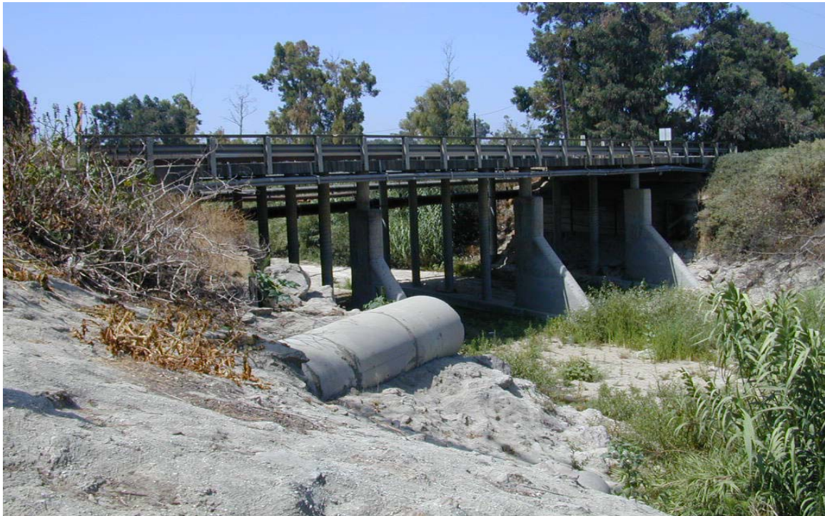
Calleguas Creek at Pleasant Valley Rd., looking downstream
