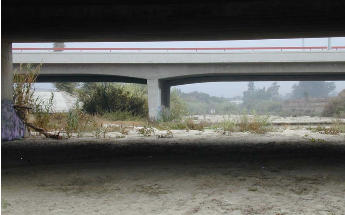
Streamgage 806 - Calleguas Creek above Highway 101 Looking Upstream
