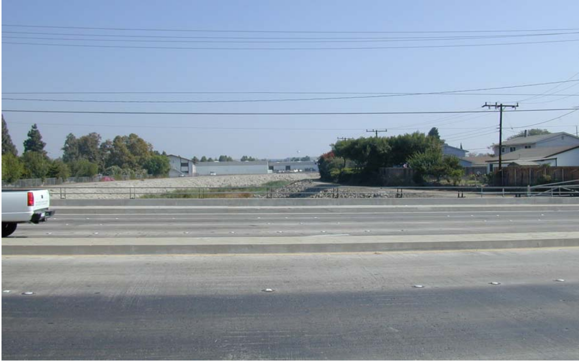
Streamgage 803 - Arroyo Simi at Madera Road Looking Upstream
