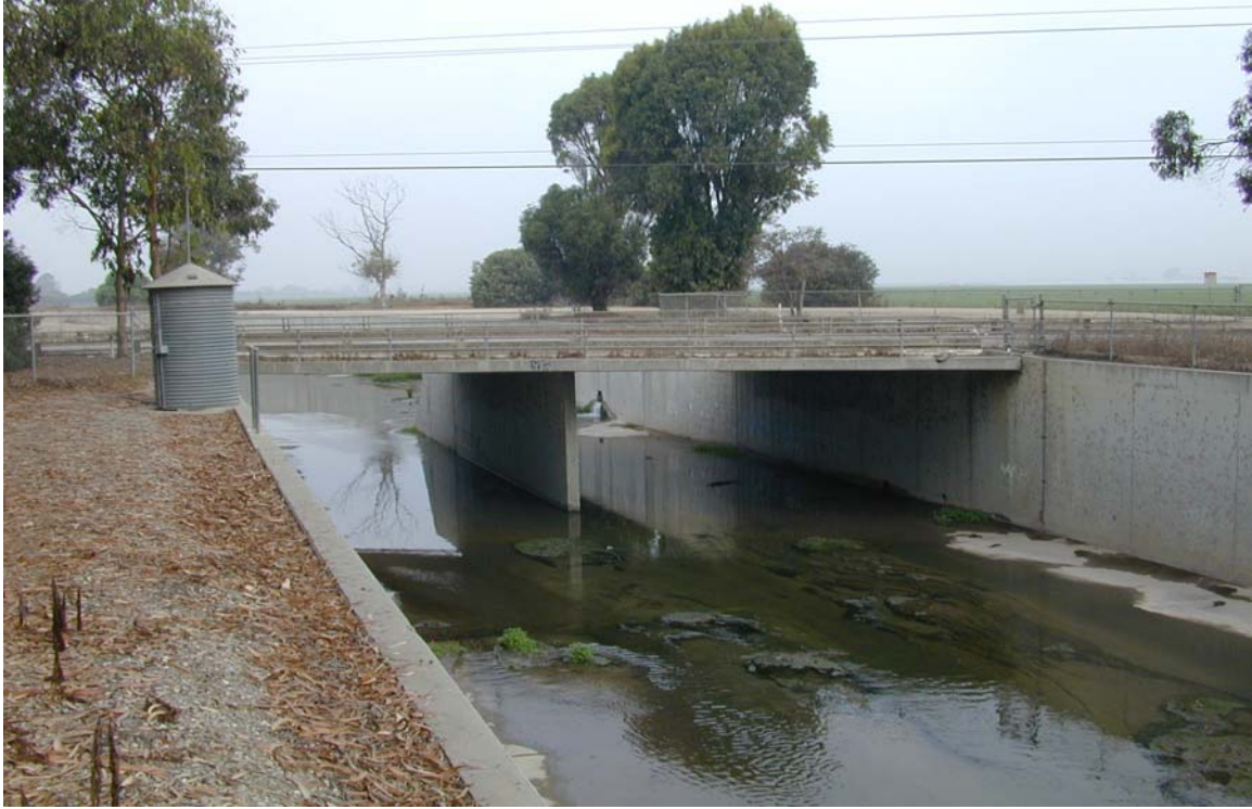
Streamgage 776 - Revolon Slough at Laguna Road Looking Upstream
