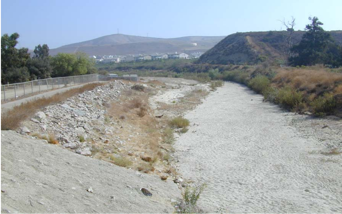
Streamgage 802 - Arroyo Simi at Royal Avenue Looking Upstream
