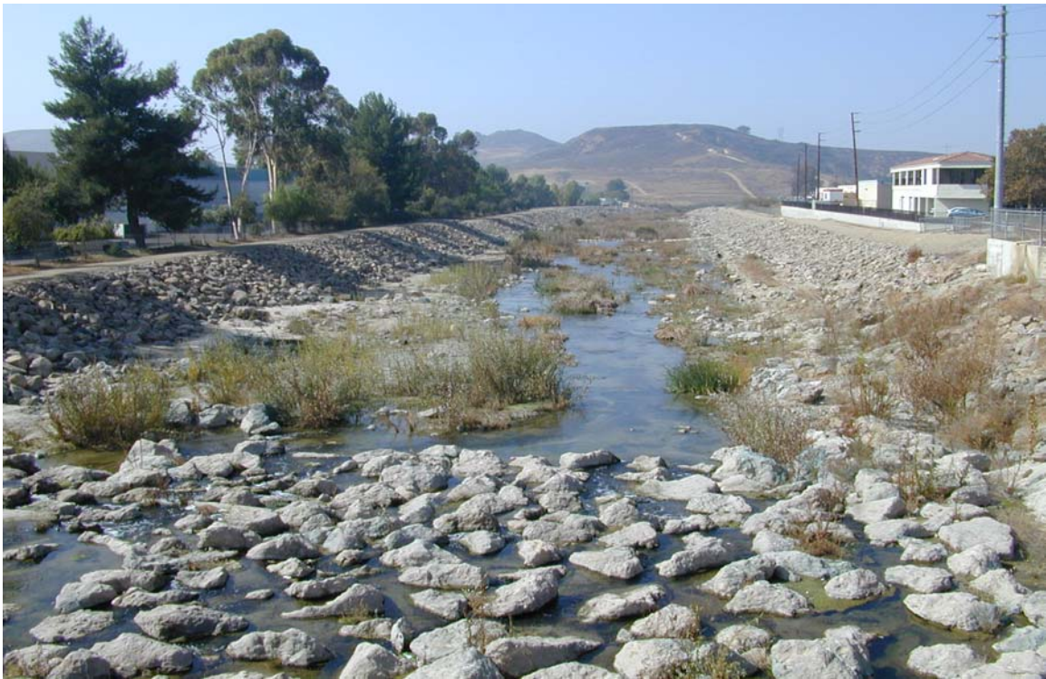
Streamgage 803 - Arroyo Simi at Madera Road Looking Downstream
