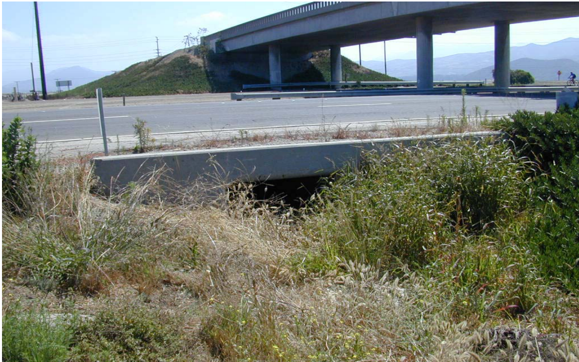
Wood Rd. Drain at PCH, looking north
