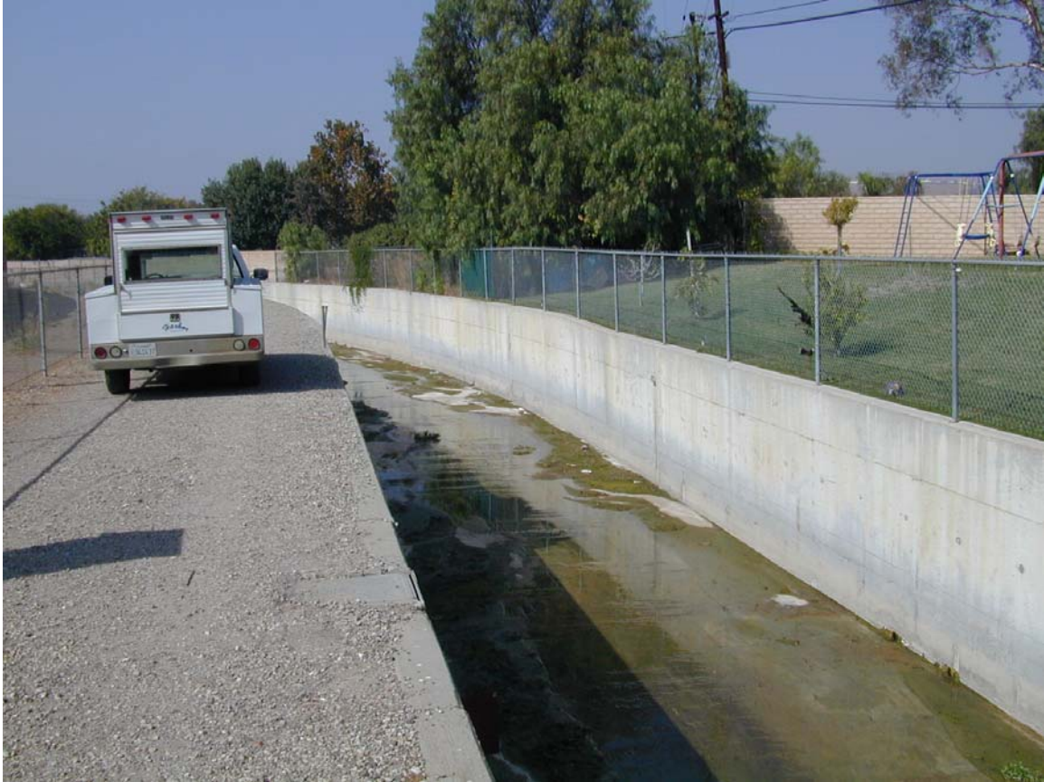
Streamgauge 831 - Arroyo Simi above White Oak Looking Downstream
