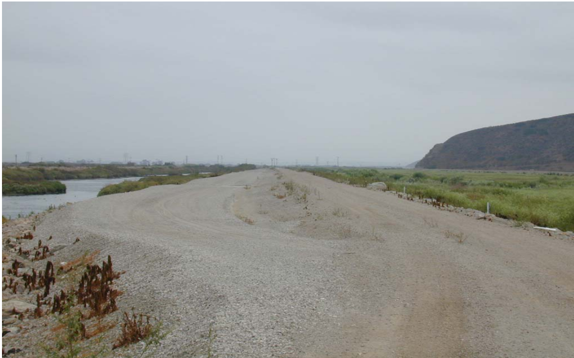
Calleguas Creek and Revolon Slough above PCH, looking upstream
