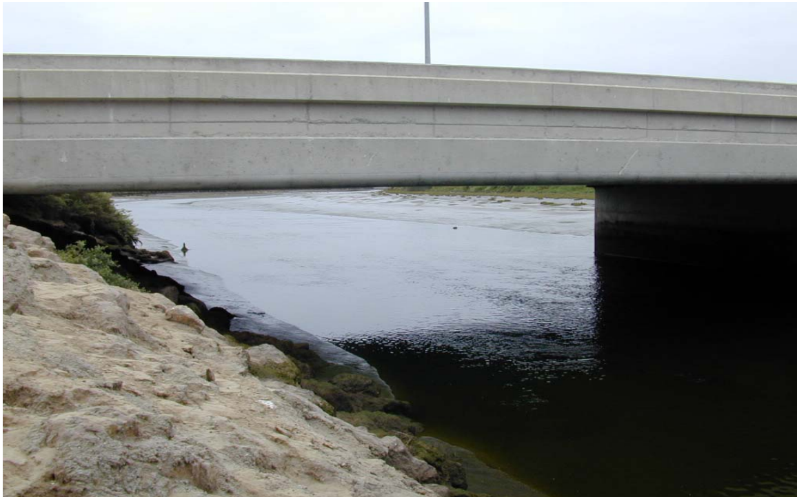
Revolon Slough at PCH, looking downstream
