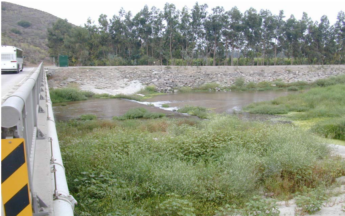
Calleguas Creek at Camarillo Dr., near CSUCI, looking downstream
