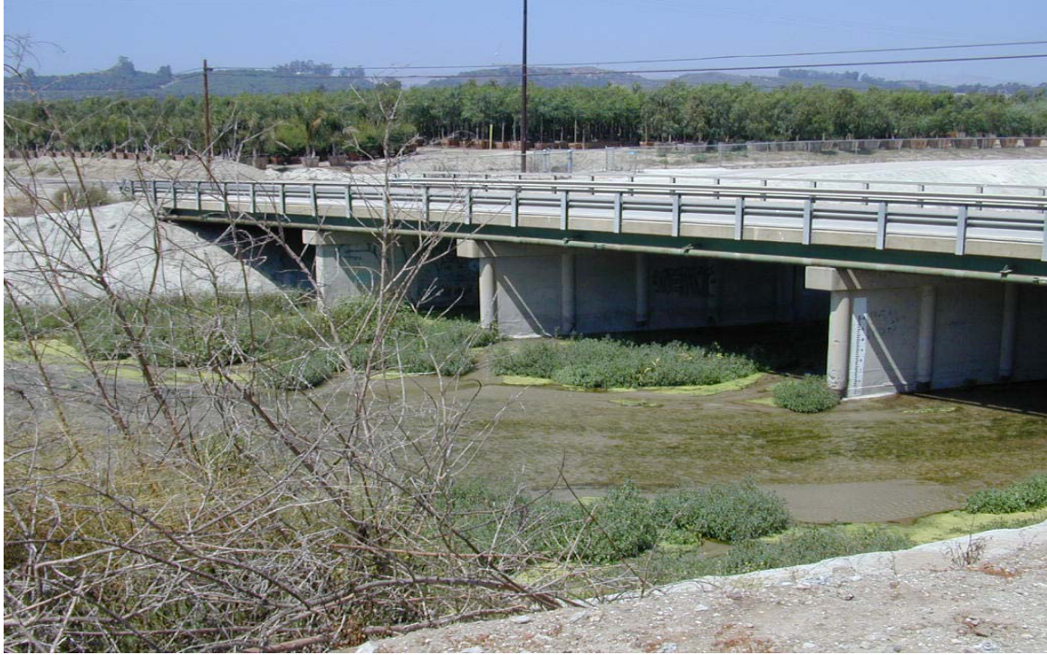
Calleguas Creek at Hitch Blvd., looking upstream
