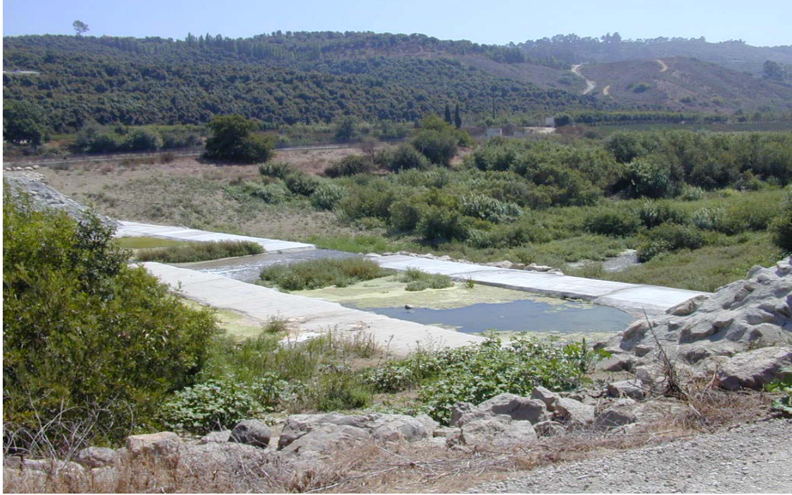
Calleguas Creek at Moorpark WWTP, looking downstream
