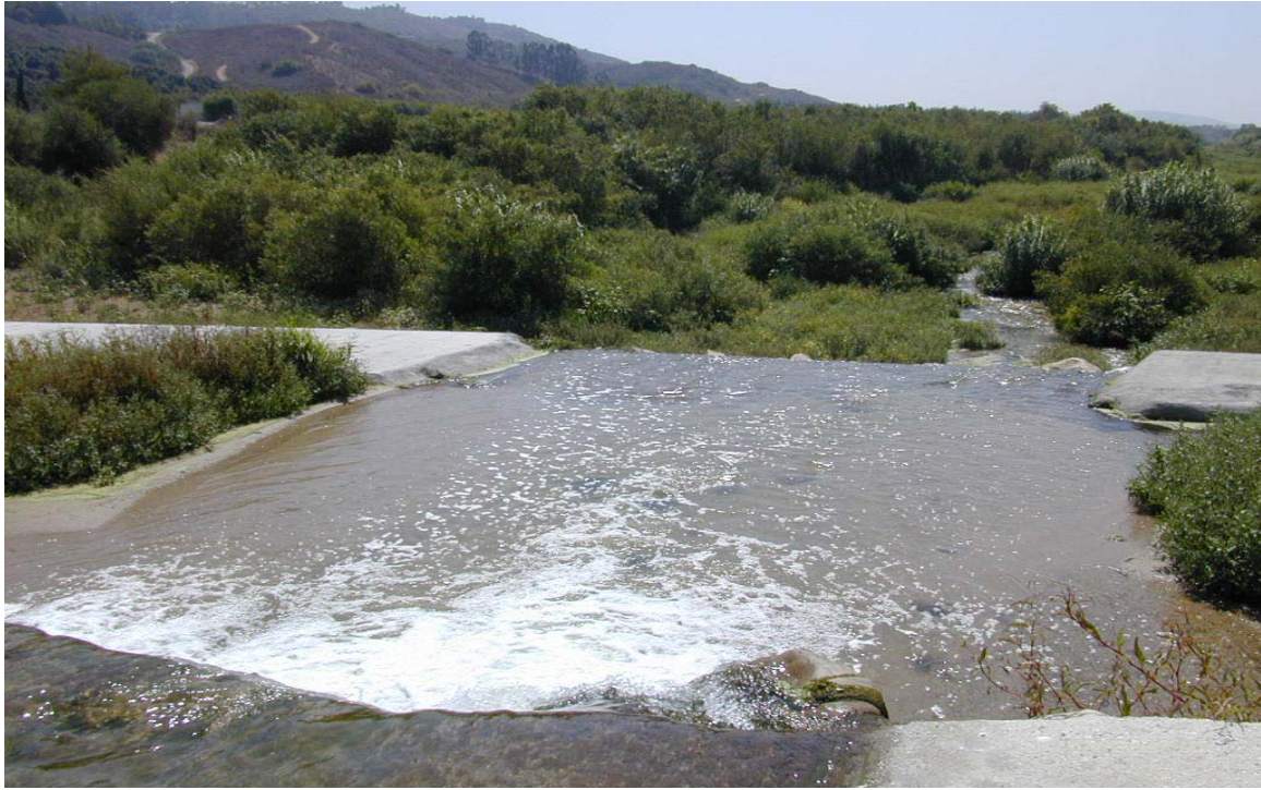
Calleguas Creek at Moorpark WWTP, looking downstream
