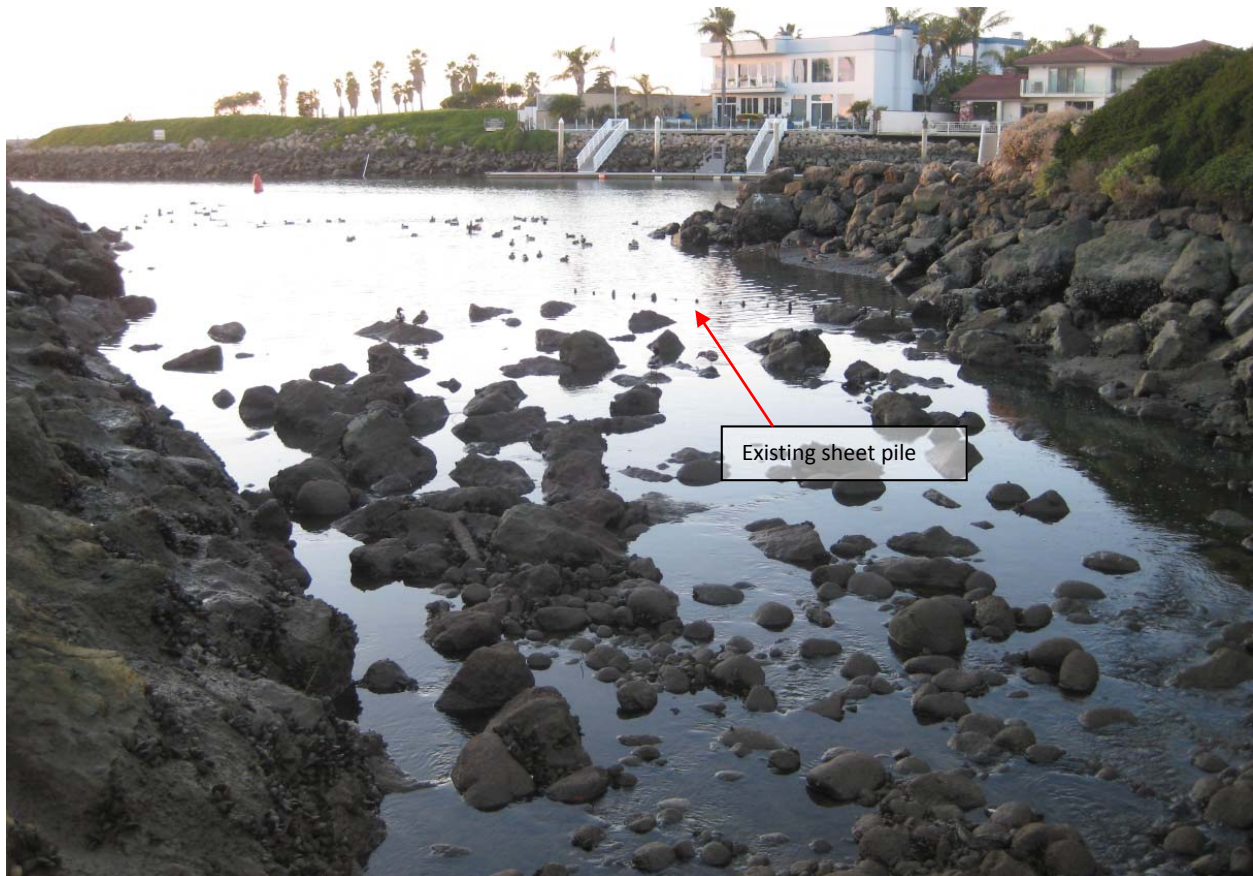
Figure 5-34. Ground view looking downstream through the Arundell Barranca outlet toward the connector channel, with the top of the sheet pile wall shown
