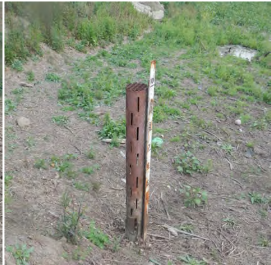
Figure 2-5. Debris Bleeder/Riser
