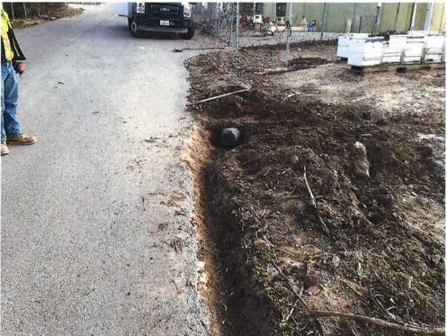
Response #4: Photos of the uncovered and screened overflow drainage line at 538 Reservoir. District 19 will make contact with the site neighbors to request the bee boxes to be relocated further away from the reservoir site. District 19 will continue to visit the reservoir site weekly to track its condition for any changes.
