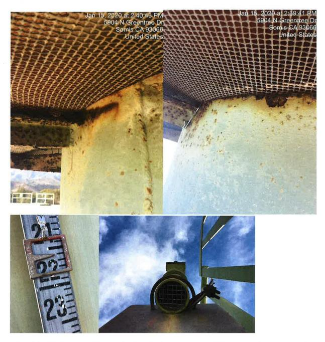
Response #6: Greentree Reservoir: Gaps in the screen around the center air vent repaired. Float indicator repaired.
