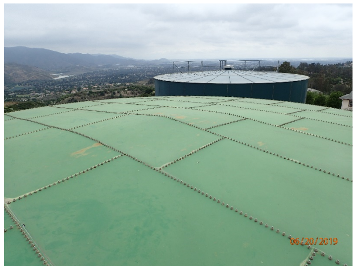
Photo 18: 860 Reservoir 1 and 2 – roofs with some paint thinning on 860 Reservoir 1.
