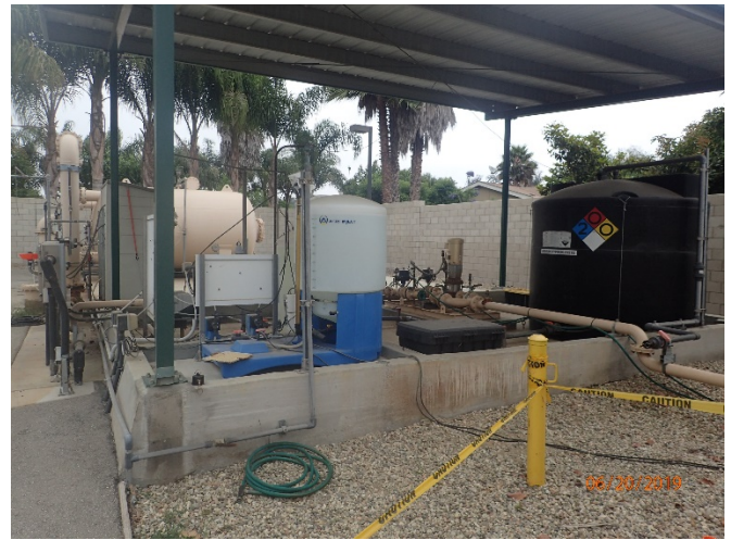
Photo 8: Well 4 treatment – chemical storage.
