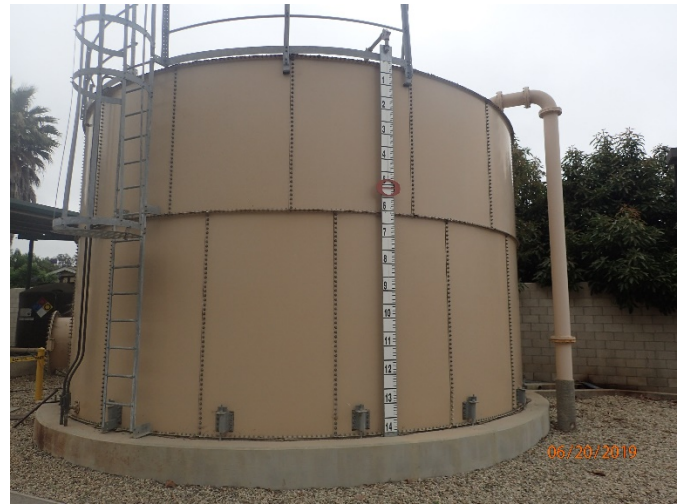
Photo 10: Well 4 treatment – backwash reclaim tank.
