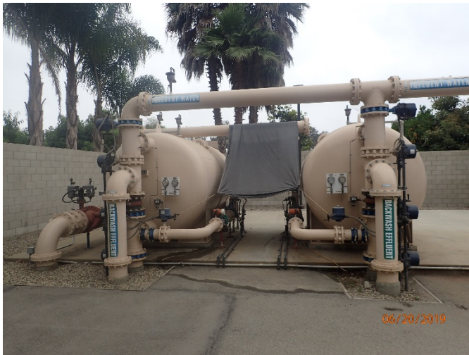
Photo 9: Well 4 treatment – pressure filter vessels.
