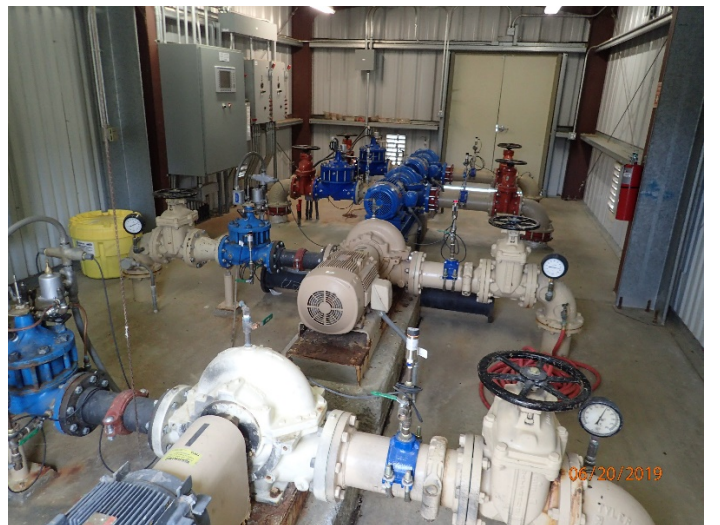
Photo 36: Sand Canyon booster pump station.
