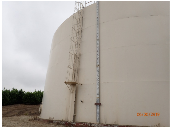
Photo 22: Balcom Canyon Reservoir (broken float level indicator).
