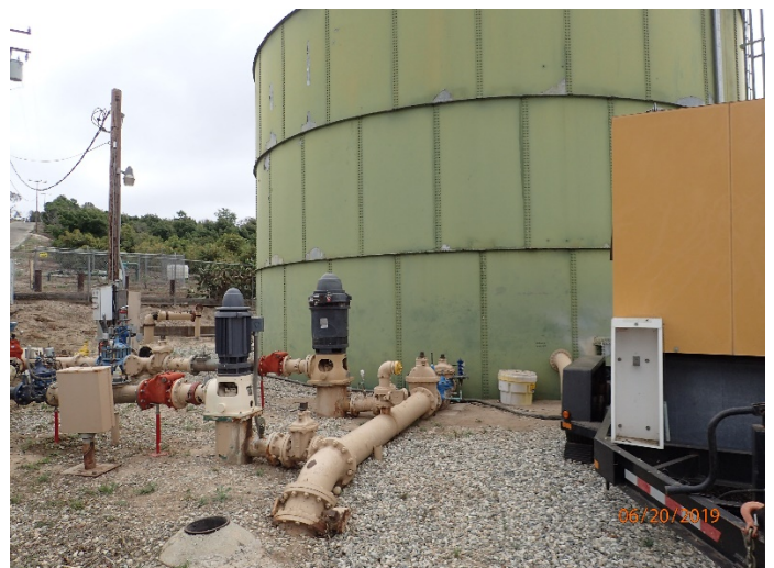
Photo 12: 538 Foot Reservoir – overview (poor paint condition).
