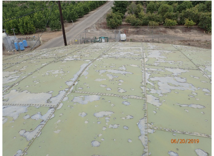
Photo 14: 538 Foot Reservoir – roof (poor paint condition; evidence of birds).
