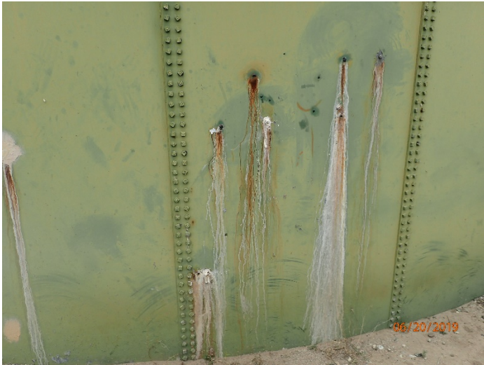
Photo 13: 538 Foot Reservoir – corrosion at previously patched spots.
