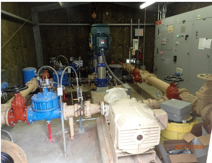
Photo 35: Greentree Reservoir 1 and 2 – housed booster pumps.
