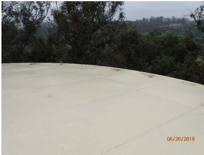
Photo 25: Balcom Canyon Reservoir – ponding on roof.
