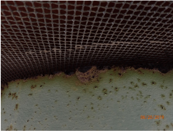
Photo 31: Greentree Reservoir 1 and 2 – gap in screen at center air vent.
