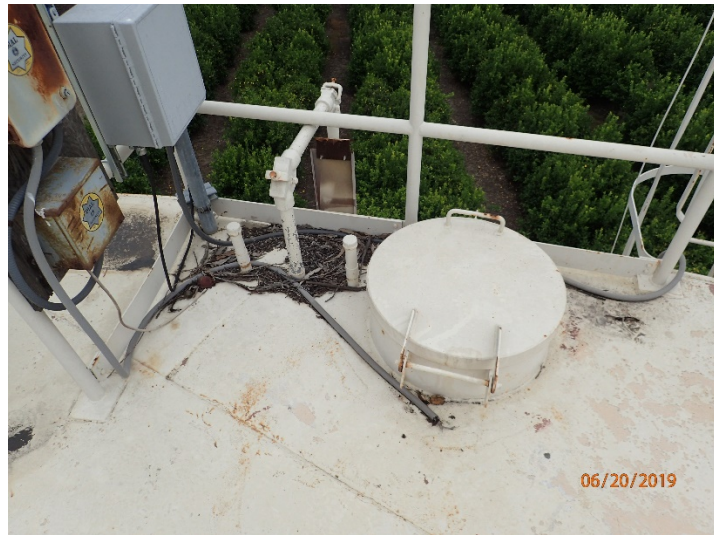
Photo 26: Balcom Canyon Reservoir – debris near hatch.
