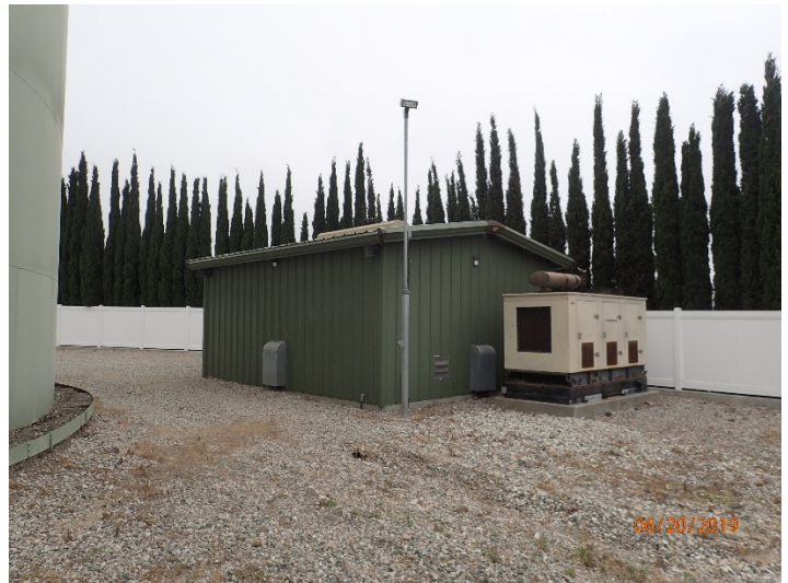
Photo 34: Greentree Reservoir 1 and 2 – backup generator and housed booster pumps.
