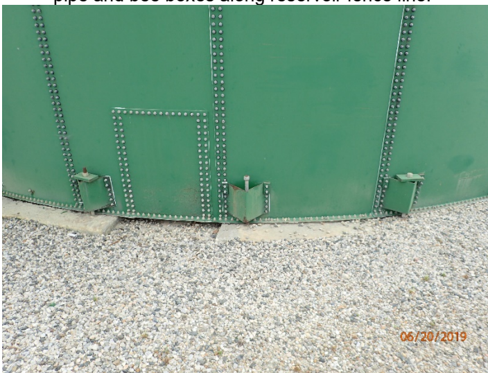
Photo 17: 860 Reservoir 1 – one tie down missing.
