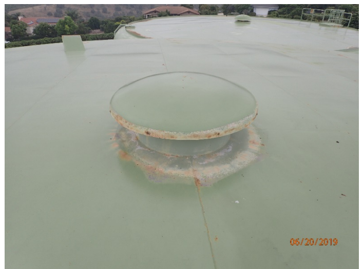
Photo 30: Greentree Reservoir 1 and 2 – roofs with corrosion where water ponds around edges.
