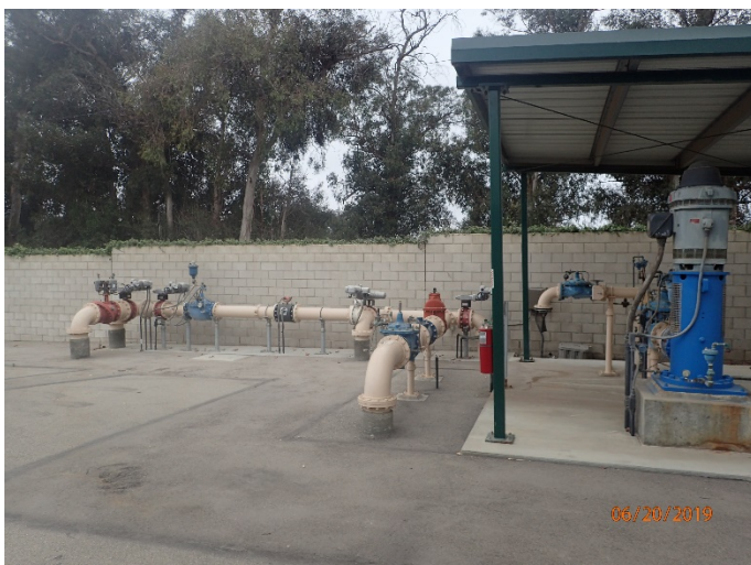
Photo 11: Booster pumps for Well 4 treated water and purchased water from Balcom Canyon turnout.
