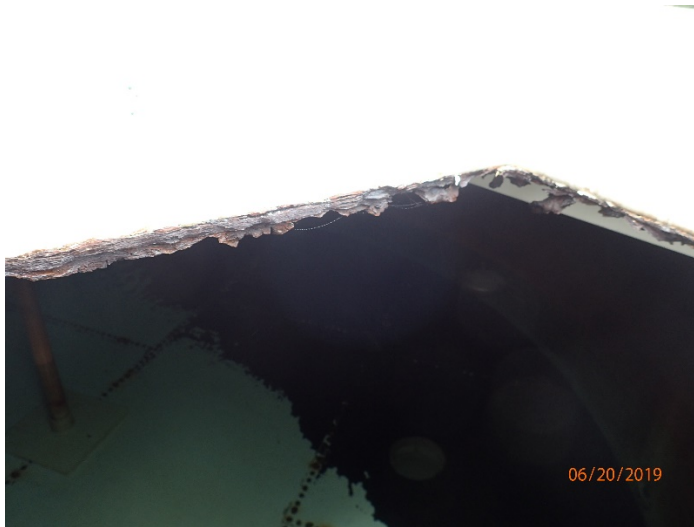
Photo 21: 1,030 Foot Reservoir 1 and 2 – interior with corrosion around edge of hatch.
