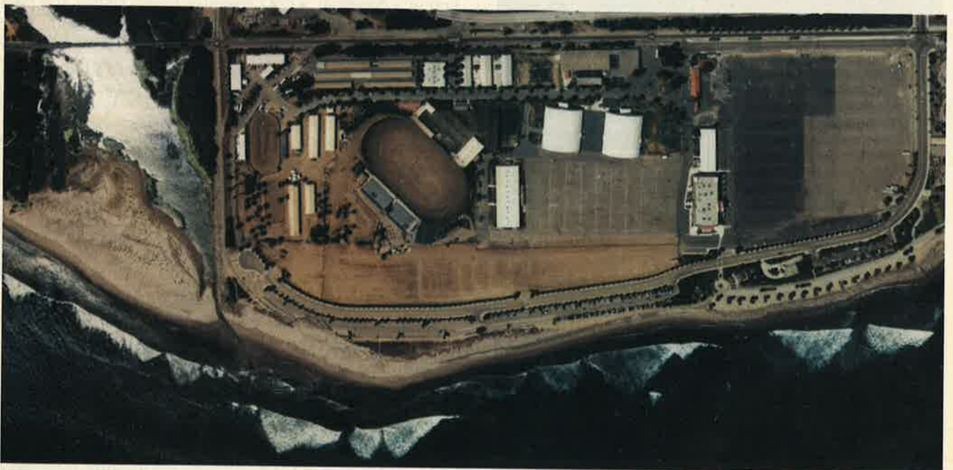
EROSION ALONG Surfers Point has wreaked havoc on a bike path and a parking facility near Seaside Park, in Ventura County, California. The Ventura River, left side of image, empties into the Pacific Ocean next to the Ventura County Fairgrounds and the park.
