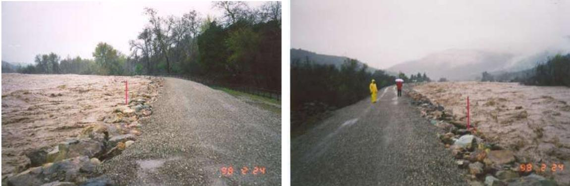
**Figure 2-24 – Upstream/Downstream Views of Casitas Springs Levee in Feb 1998 Storm Event (<20 Year Event)**
