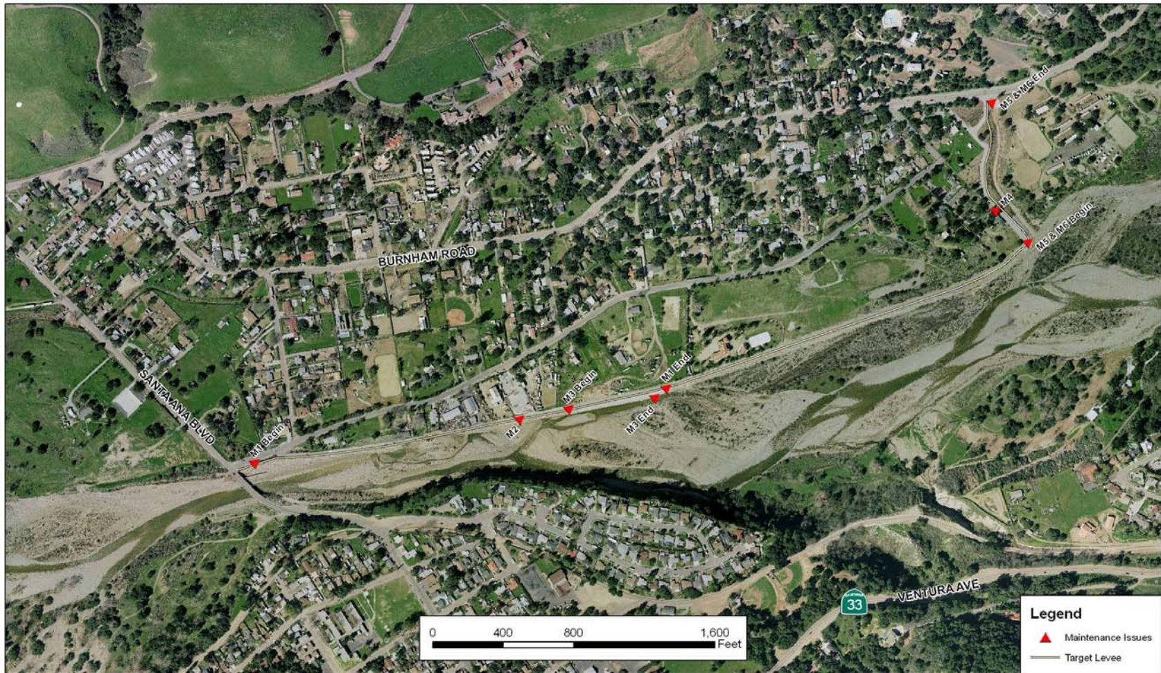
Appendix C – Photograph Locations of Maintenance Required Areas along Ventura River Levee and Floodwall (VR-3)
