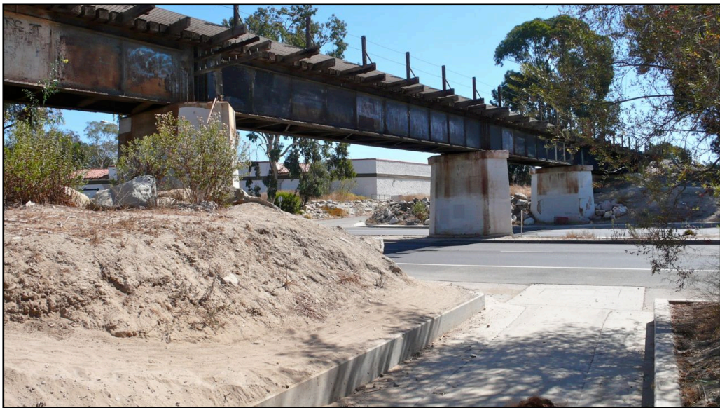
Photo 3. Ventura Road crossing, western side, view towards southeast. [9-18-2014]
