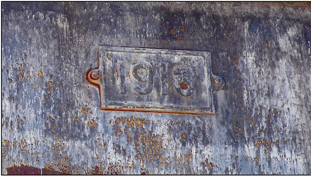
Photo 7. Date of construction plaque, second span, western side. [9-18-2014]
