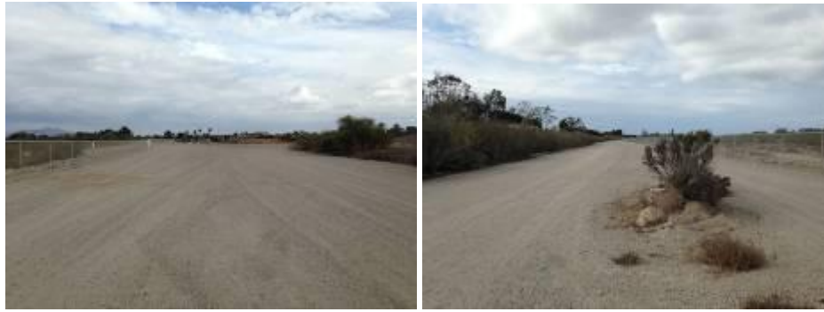
#15-16- Facing NE and SW- At the start of Reach 3
