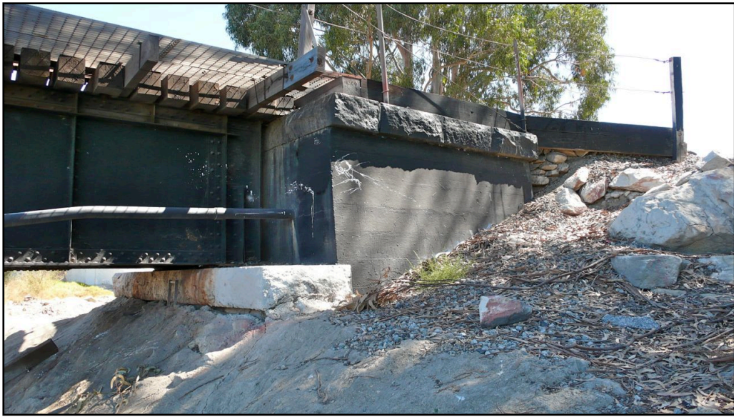
Photo 4. Southern abutment, western side. [9-18-2014]
