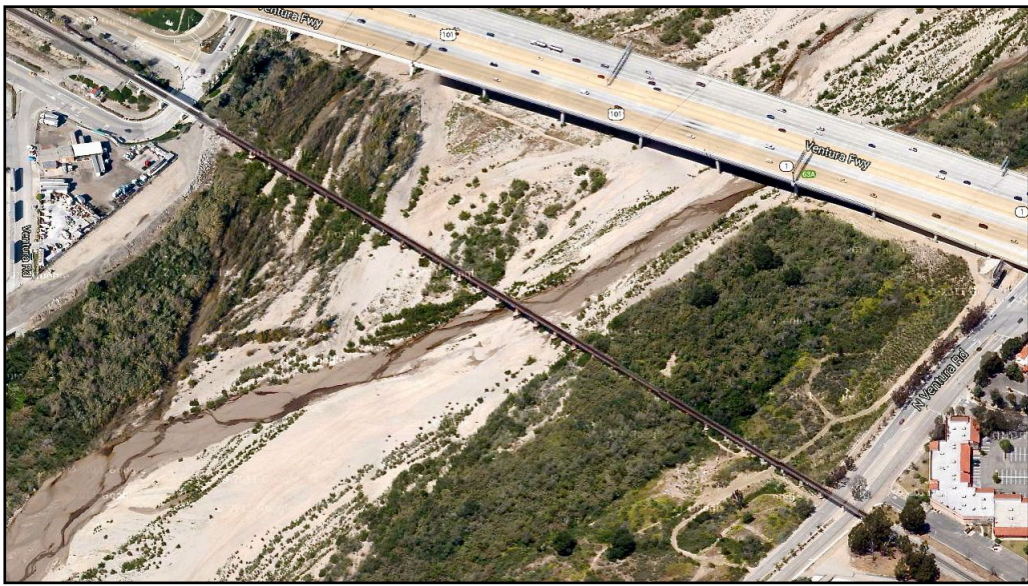
Photo 1. Oblique aerial, view from south. [Google Maps, nd]
