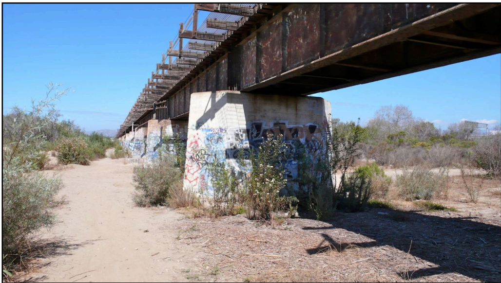
Photo 2. Railroad trestle within riverbed, downstream side, view towards north. [9-18-2014]
