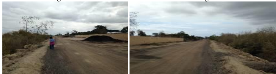
Facing E and W- At the end of Reach 2
