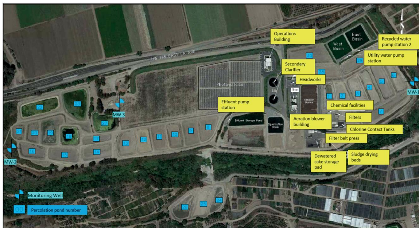
Figure 1-2: Moorpark Water Reclamation Facility Aerial View
