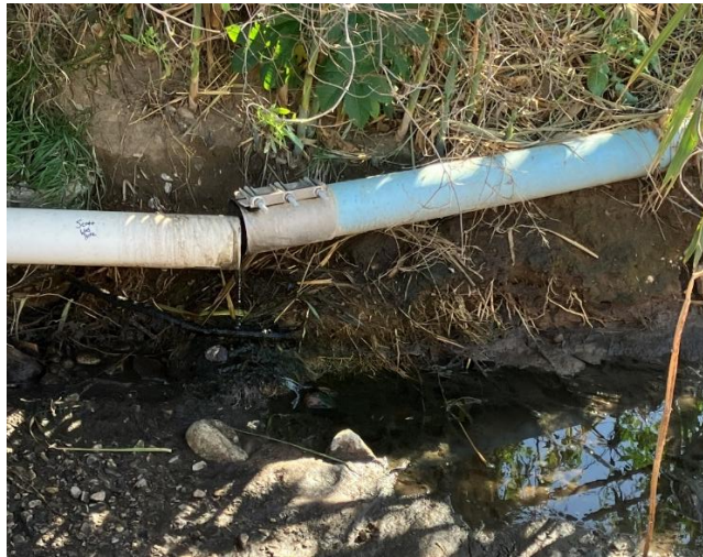
Figure 3-13: Separated Sections of Effluent Piping
