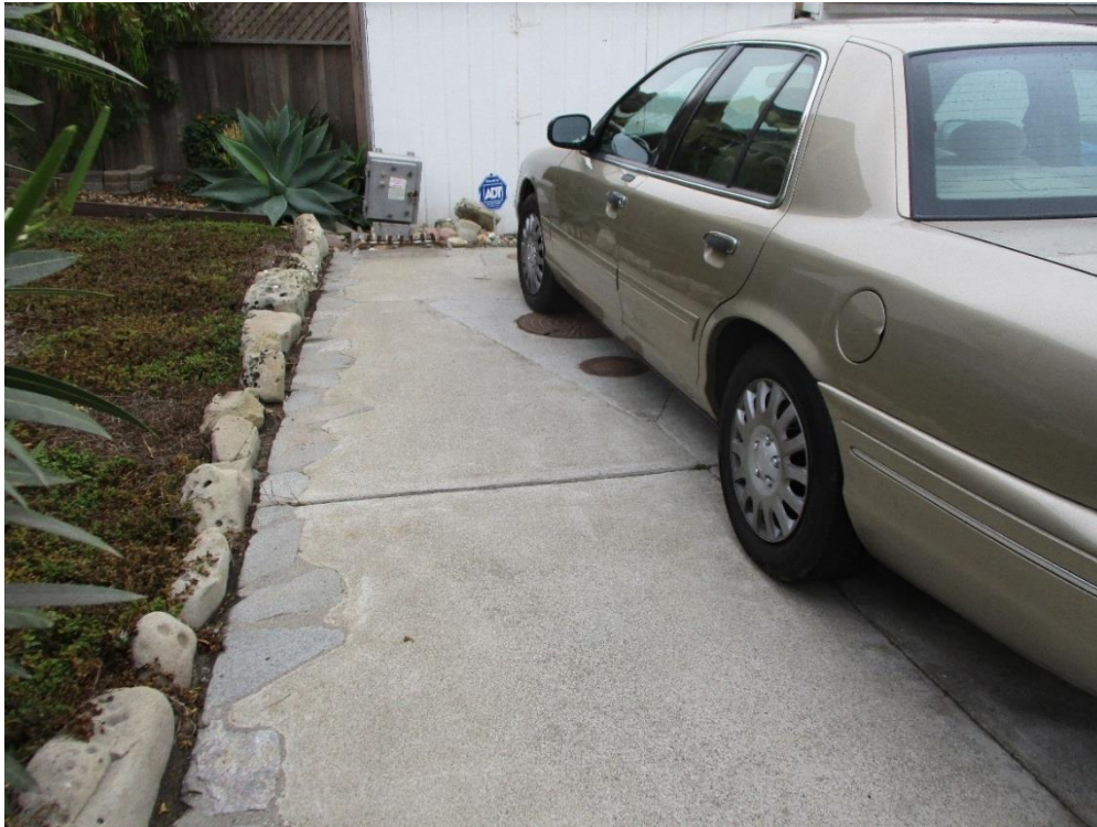
Example of Tank Access Issue due to Vehicles
