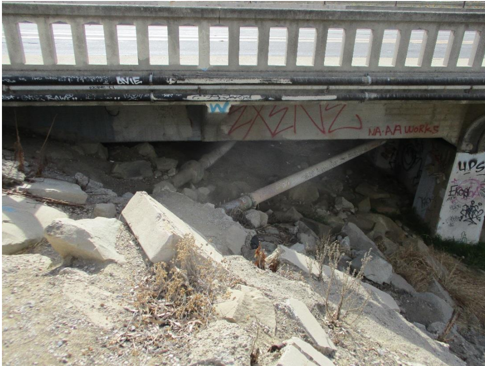
Force Main Piping Exposed on Left – No Protection
