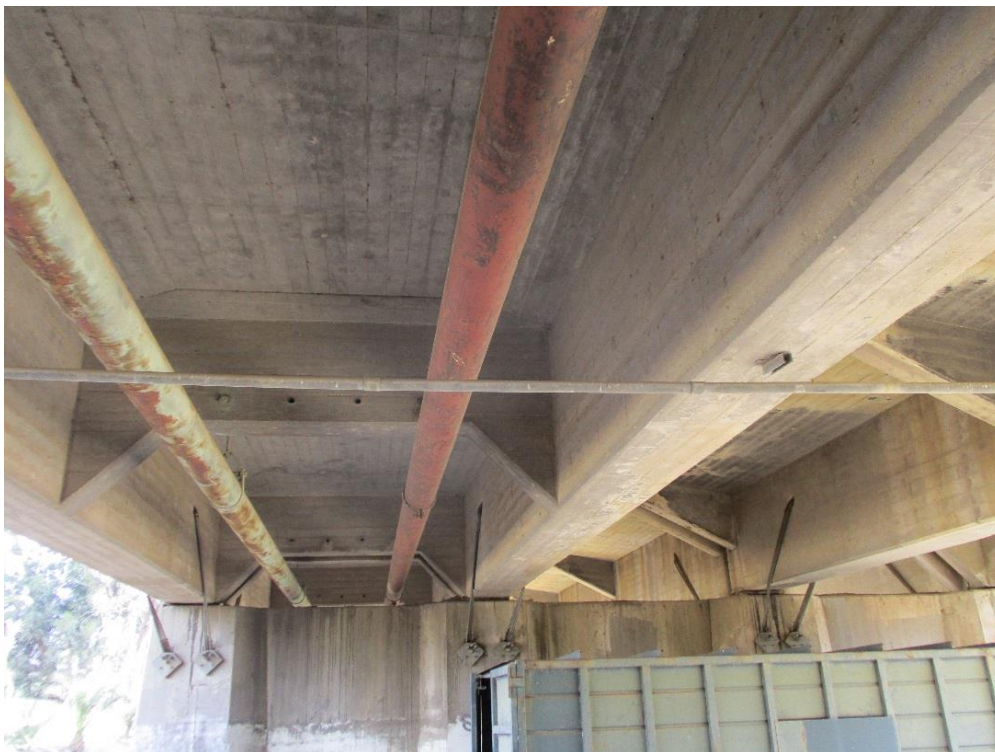
Force Main Piping Exposed Under Bridge (Right Side)
