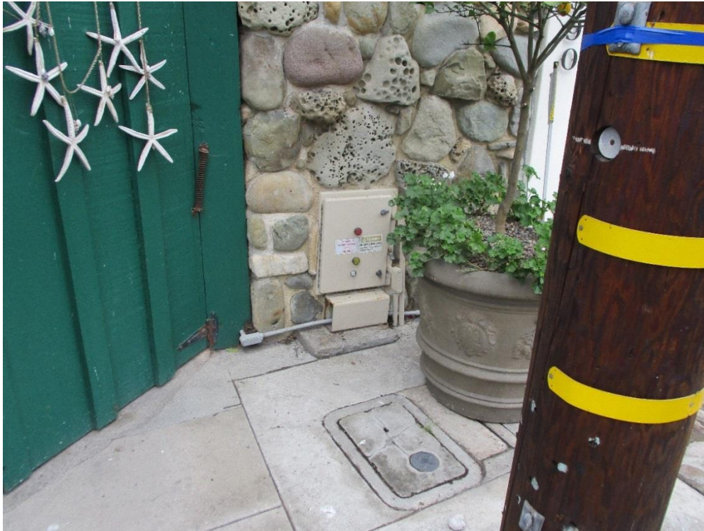
Control Panel Cast into Block Fence
