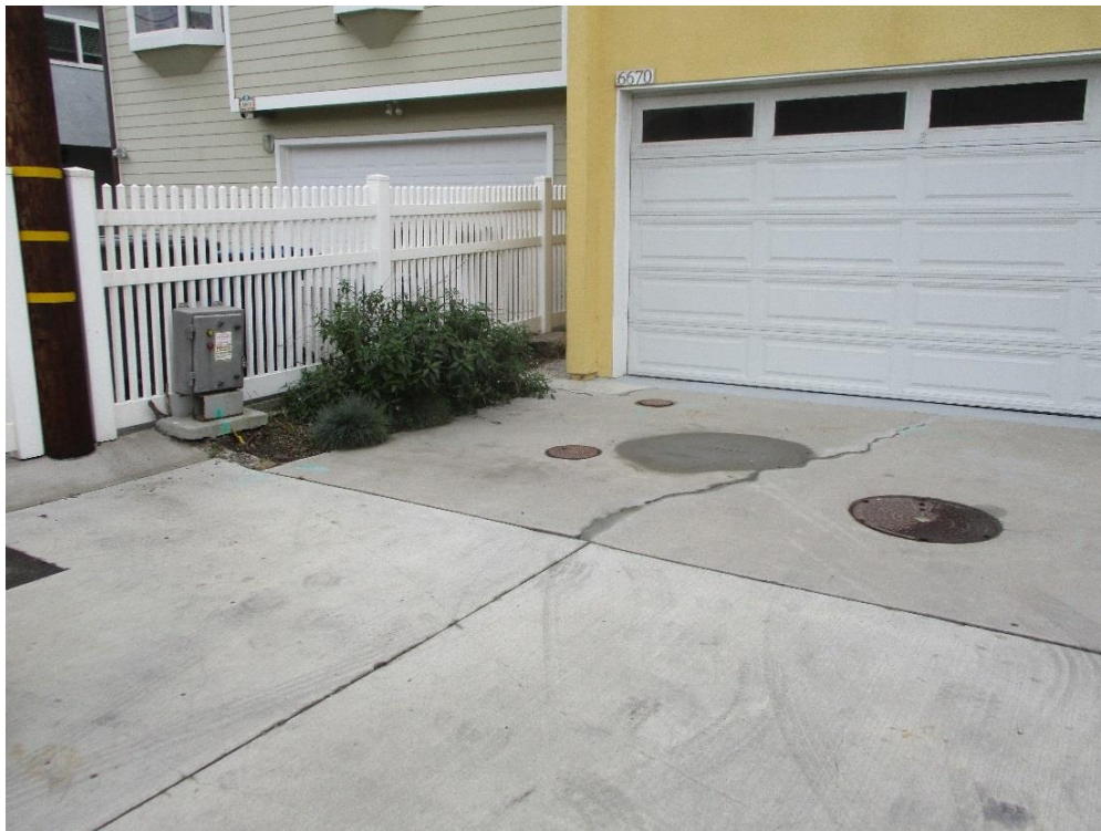
Typical Control Panel and Tank Configuration – Driveway
