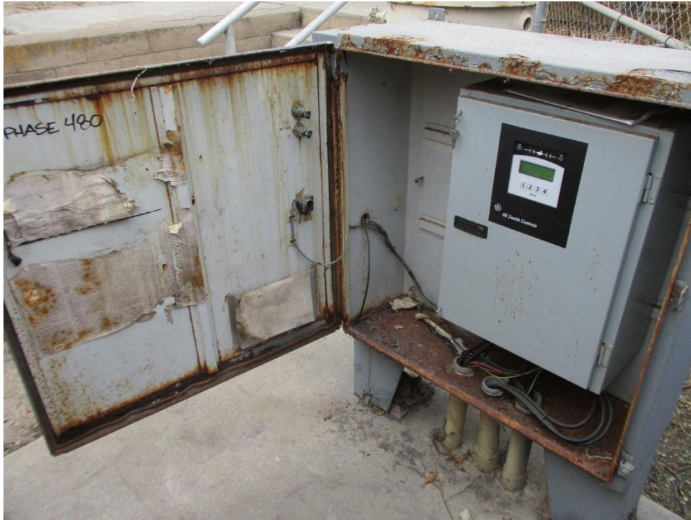
Control Panel Interior at Seacliff Lift Station
