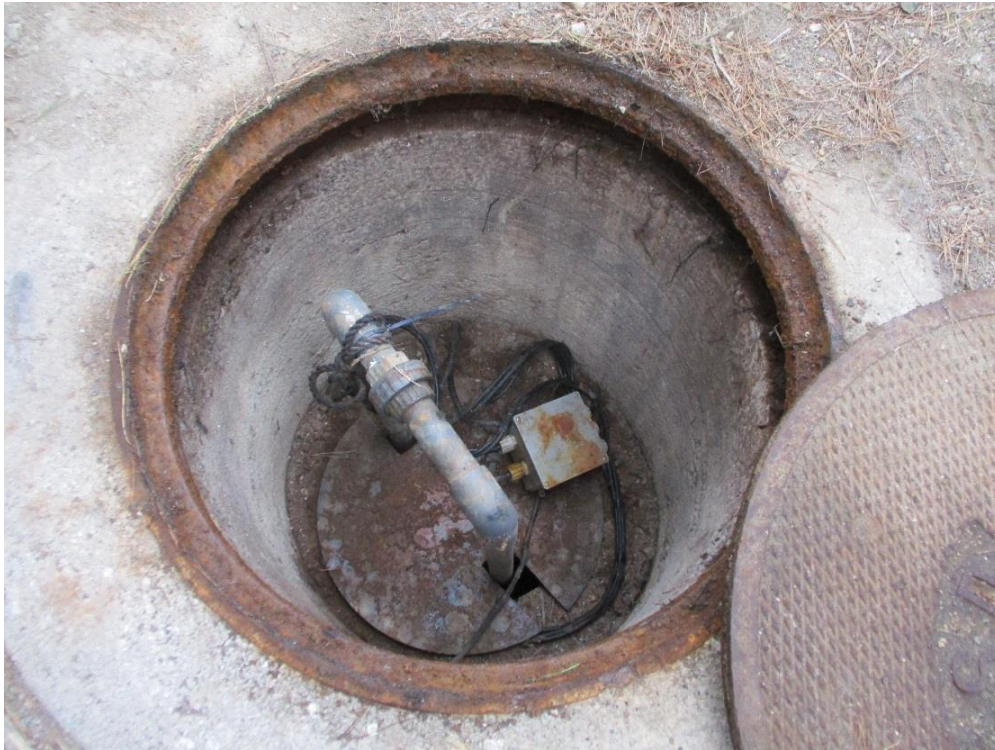
Typical Interceptor Tank Interior Configuration From Above
