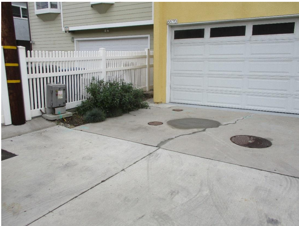
Typical Control Panel and Tank Configuration
