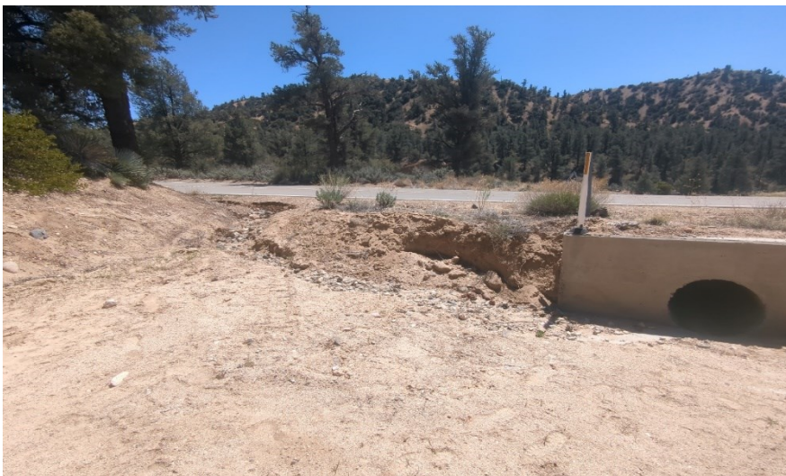
Photograph 9. View of Unnamed Drainage 2 joining Unnamed Drainage 1 in the MP 12.69 project site, facing southeast (April 23, 2025).
