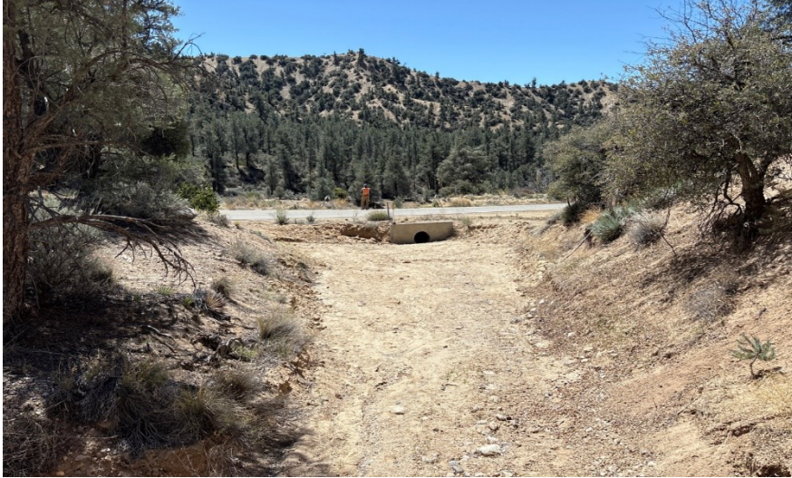
Photograph 7. View of Unnamed Drainage 1 at the MP 12.69 BSA, facing south (April 23, 2025).
