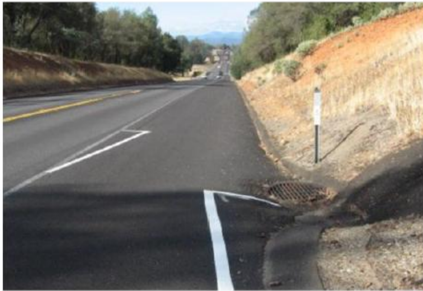
California State Route 44 in Shasta County, California. The painted “Flying Wedge” alerts bicyclists to a drainage grate and the beginning of a rumble strip.
