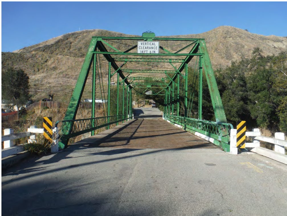
Figure 15. Overview of County Bridge #442; Caltrans Bridge #52C-0053, view west.
