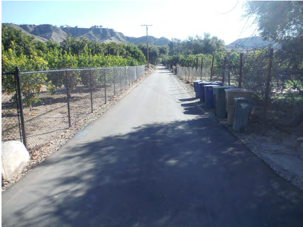
Figure 18. Overview of the Bridge Road access portion of the APE, view south.
