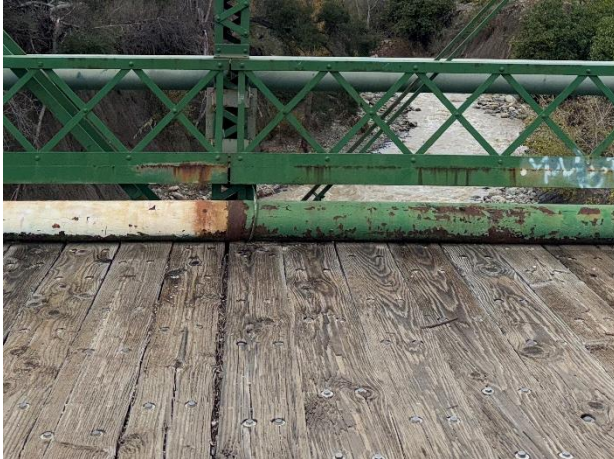
Figure 4. Detail of wood timber deck (GPA, 2026).
