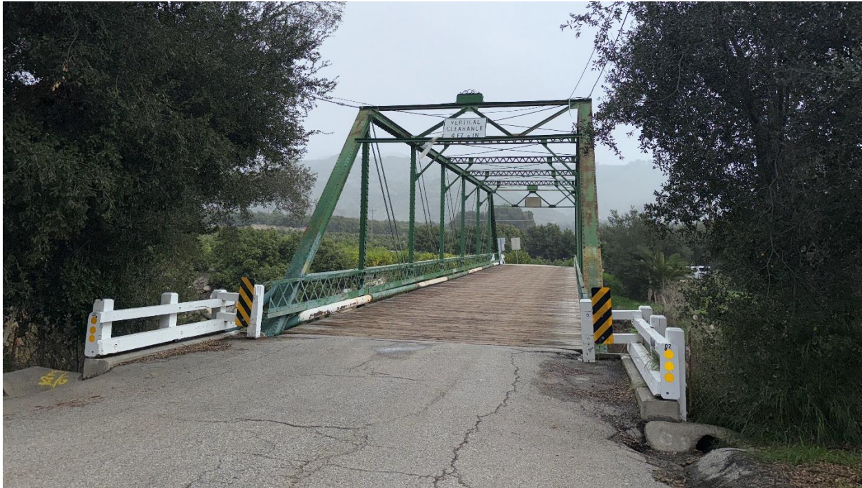
Figure 2. View of Bridge Road Bridge looking east (GPA, 2021).
