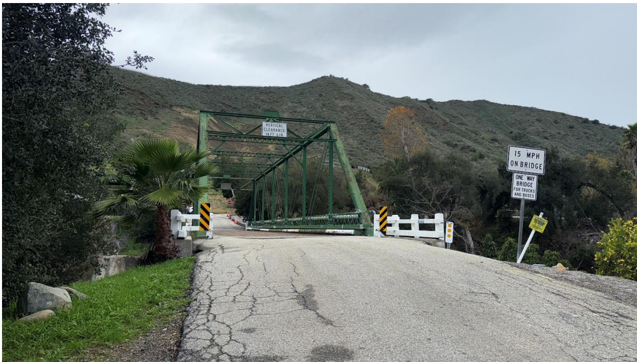
Figure 3. View of Bridge Road Bridge looking west (GPA, 2026).
